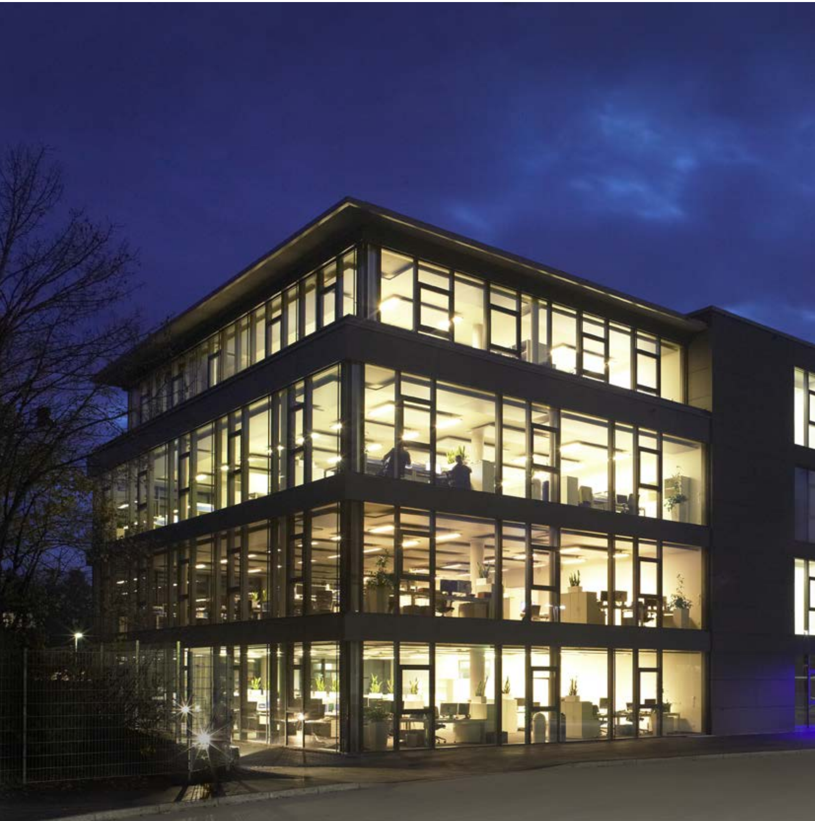
Administrative building of BHS-Sonthofen
