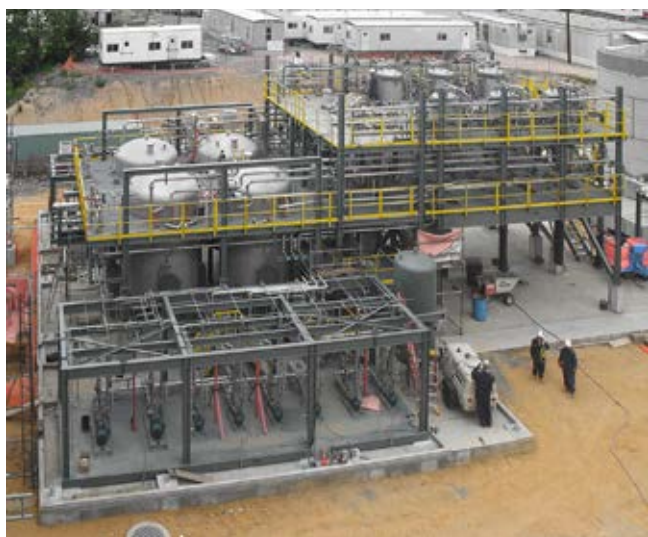
In a North American refinery, catalyst particles are extracted by a gas scrubber and cleaned by means of two BHS candle filter plants operating in parallel. Each plant contains two BHS candle filters of type CF 24-147, each with 100 m 2 filter area, and a precoat plant.
