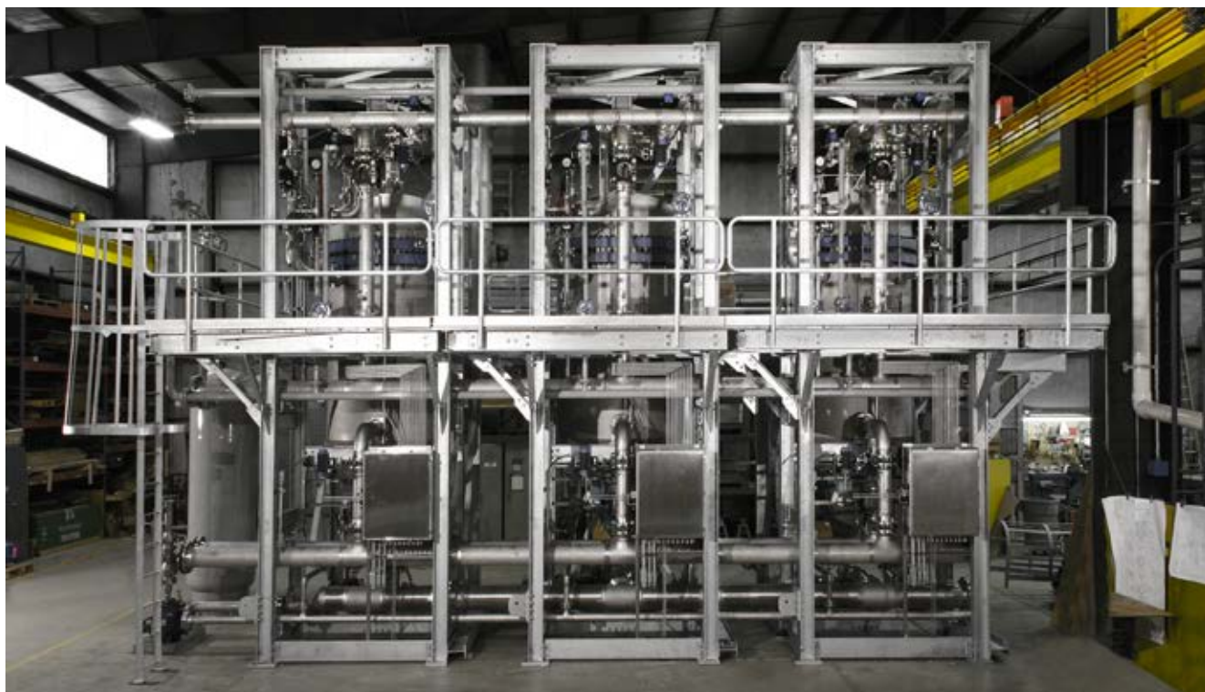
The BHS candle filter plant of type CF 179-66 consists of three identical candle filters, each with 66 m 2 filter area, and is used for gray-water regeneration in a coal-to-gas plant.
