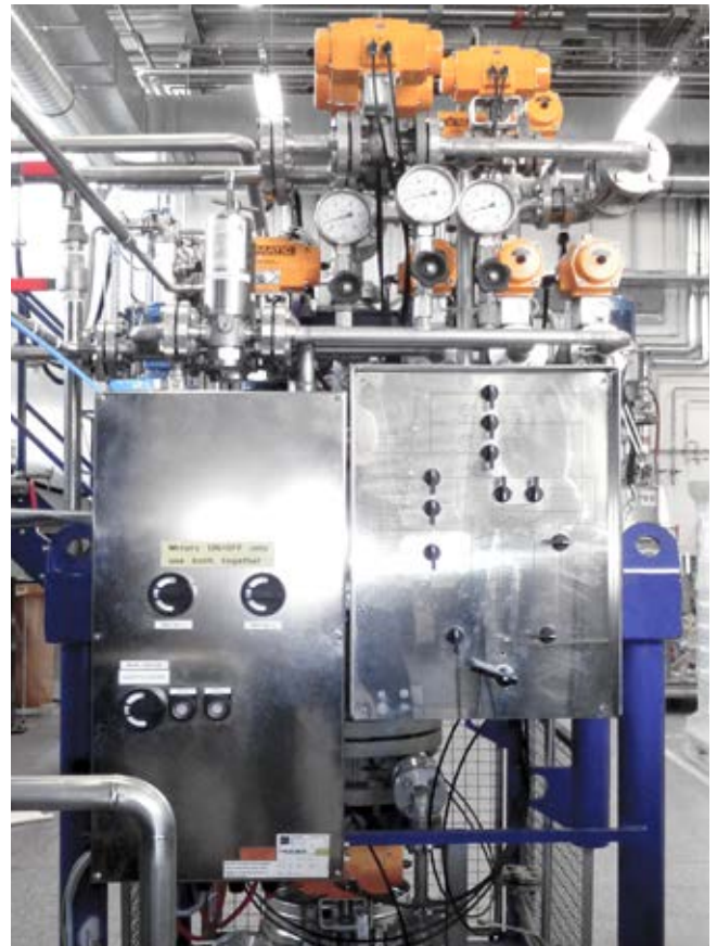
System controller for the pilot plate filter skid
