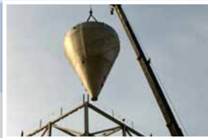
Large capacity spray drying plant installation. Spray dryer delivered to site in sections for final fabrication.
