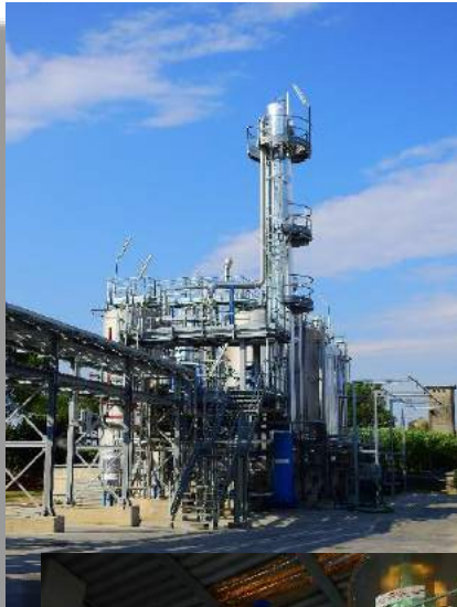
« Distillation + Concentrator + Evaporator » project in Italy Status: In operation
